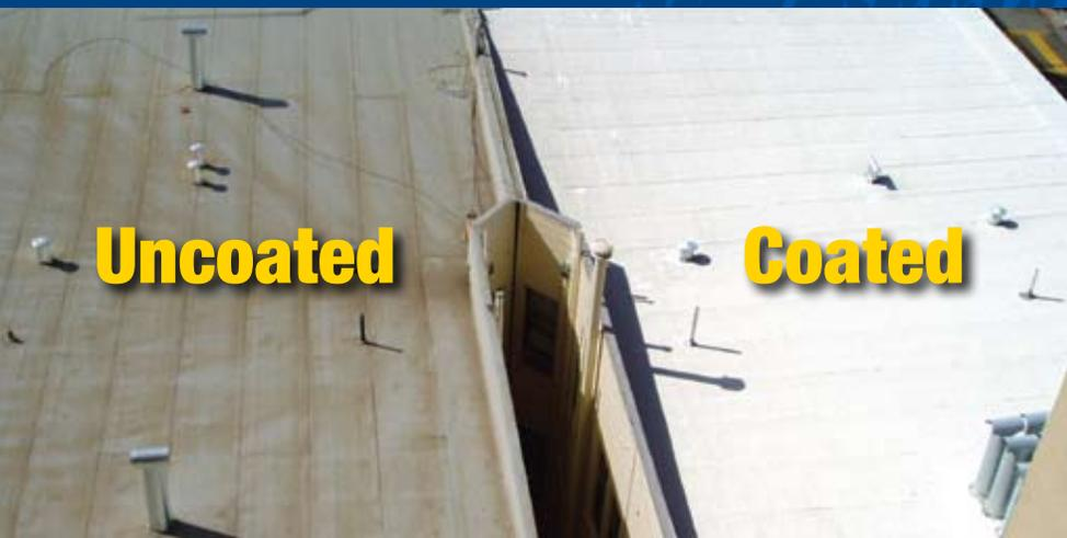
**ENERGY STAR compliant Henry white roof coatings can significantly reduce the energy costs required to keep a building or home cool.**
