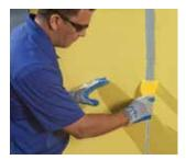
**Air-Bloc LF** is a liquid-applied, single-component, high-solids, Silyl-Terminated—Poly-Ether (STPE) that is easy to gun, spread and tool. Importantly, Air-Bloc LF provides best-in-class compatibility with asphalt, which is critical to a long-lasting, successful wall design. Air-Bloc LF can be left exposed for six months and, once cured, results in a permeable, durable and seamless flashing membrane with excellent weathering, water resistance and nail sealability (meets AAMA 711).
