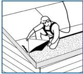
Remove nails. Apply sealant to rake; release film from the upper portion and adhere in place.
