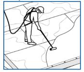
Install metal drip edge at rake and eave. Apply primer by roller or pump-up sprayer at a rate of approx. 300 ft²/gal. (28 m²/3.78 L). Allow to dry.
